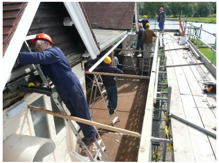
New tanilised timber is secured to the tops of the window frames to provide rigidity and a base for the new aluminium roofing bar system.
