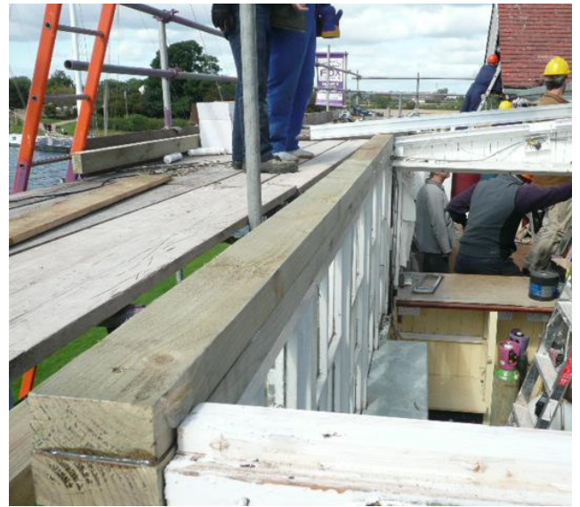
By lunchtime the new timber is in place and the horizontal glazing support sections have been half fitted. Roger works on lining up the first glazing panel while the bar roof Conga gets going
