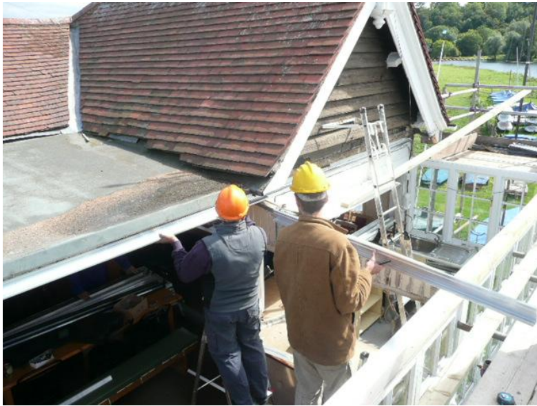
New tanilised timber is secured to the tops of the window frames to provide rigidity and a base for the new aluminium roofing bar system.
