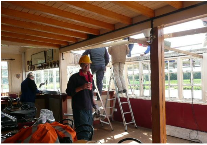
New tanilised timber is secured to the tops of the window frames to provide rigidity and a base for the new aluminium roofing bar system.
