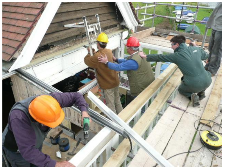
By lunchtime the new timber is in place and the horizontal glazing support sections have been half fitted. Roger works on lining up the first glazing panel while the bar roof Conga gets going
