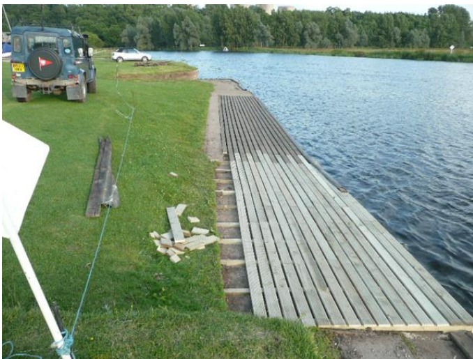
Old staging is removed and replaced with tanilised decking
