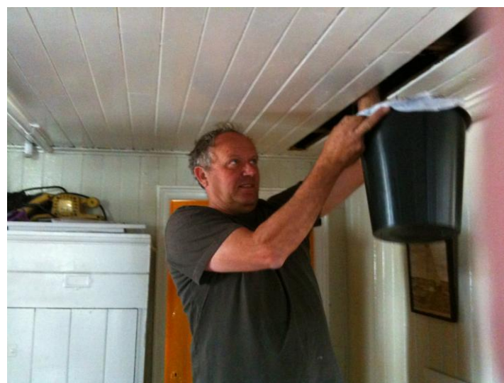
Clearing the middle ceiling void
