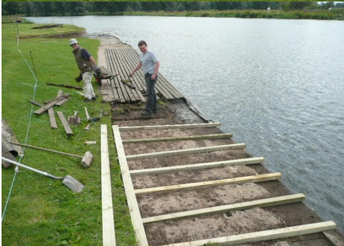
Old staging is removed and replaced with tanilised decking
